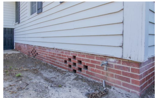
Figure 13 Typical Ford-era brick foundation on Ford Avenue.
