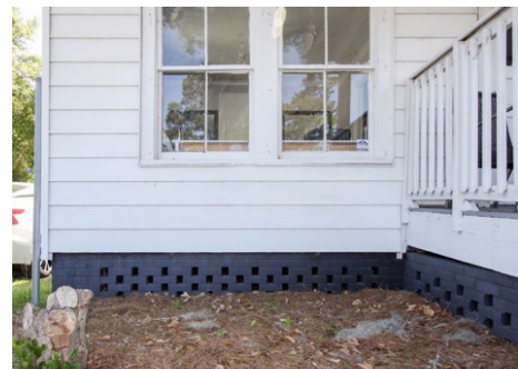
Figure 16 A historic brick foundation that has been painted.
