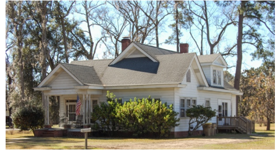
Figure 27 An image of the Mitchum House illustrating the use of asphalt shingle roofing.
