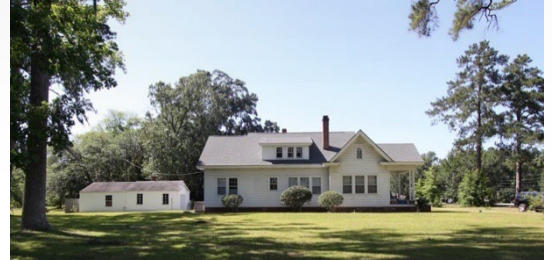
Figure 36 The Mitchum House and garage, which sits at the rear of the property, detached from the main house.
