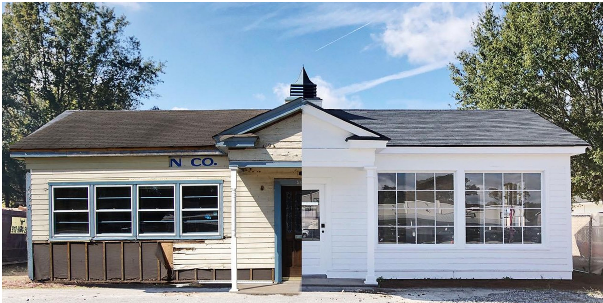
Figure 11 The Ford Bakery before and after rehabilitation.
