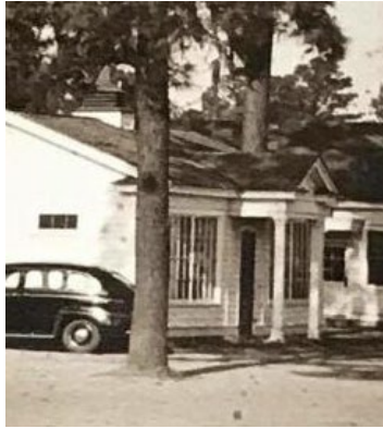
Figure 19 Before, historic, and after images of the windows at the Ford Bakery showcasing the utilization of historic imagery to recreate missing features.
