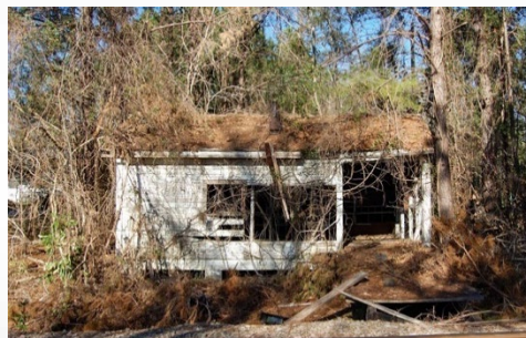
Figure 32 Railroad Postal Delivery Building.
