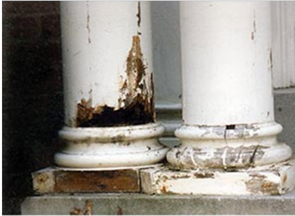
Figure 23 Before and after images of deteriorated wood column bases which have been repaired following the removal of the deteriorated sections, reusing as much historic material as possible.
