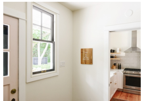
Figure 20 An interior storm window, shown in black, paired with a historic double hung sash.
