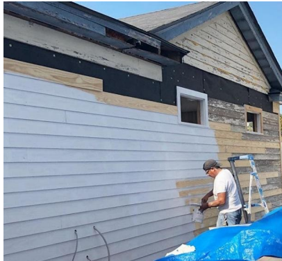
Figure 15 Wood siding repair and replacement and subsequent painting at the Ford Bakery.
