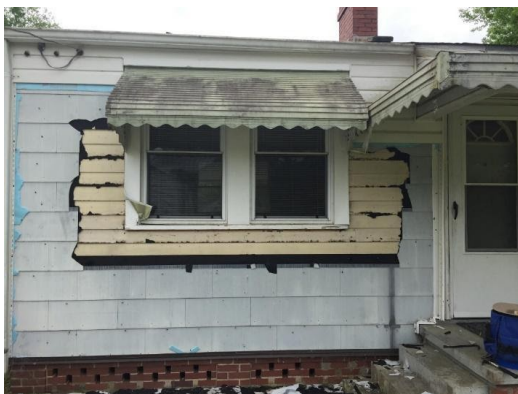
Figure 17 Historic wood siding revealed during the removal of vinyl and asbestos shingle siding.
