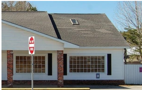
Figure 28 A skylight placed on the front facade of a historic building.
